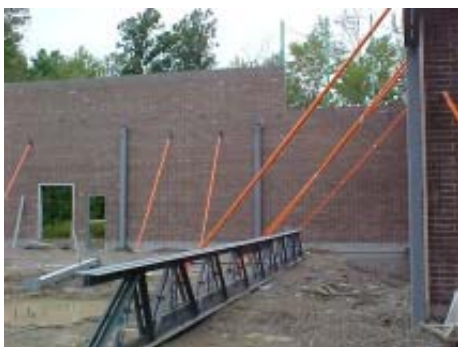
Photos: Crowe Masonry Jobsite
